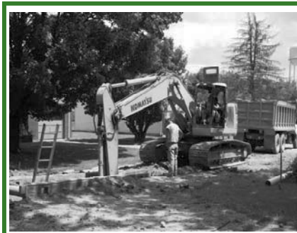
Field's Excavating works on Walnut Street in Brandt.
