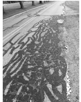
Crack Sealing can extend the life of a road. Many of our roads have extensive crack sealing on them.
